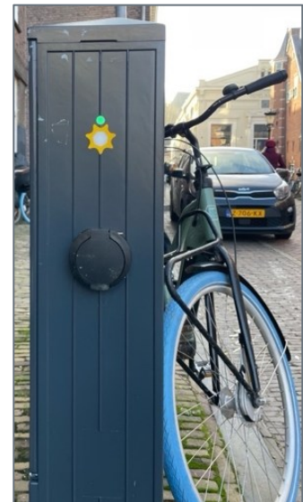
Figure 1: LomboxNet AC-V2G EV charging post, Utrecht. Post has two power outlets and can charge/discharge (in any combination) two cars simultaneously at 7kW.
